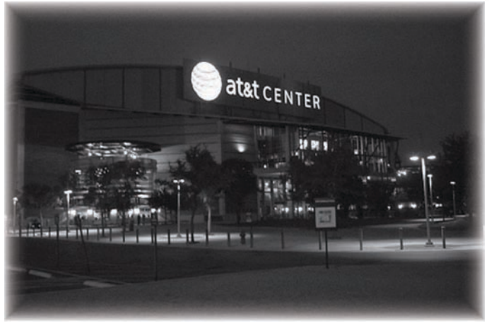
The AT&T Center is the home to the San Antonio Spurs and San Antonio Silver Stars.
