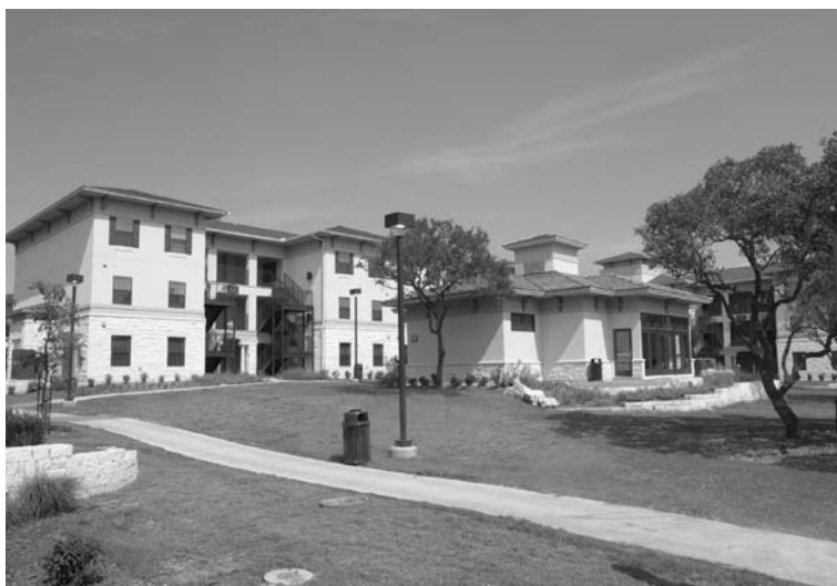
Chaparral Village opened in 2004 and houses more than 1,000 students.
